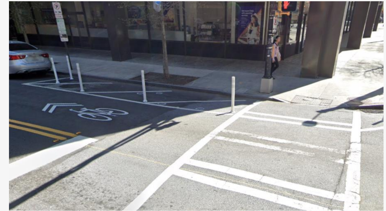
Painted and buffered bulb-outs/curb extensions on Dill Ave around AMP.
