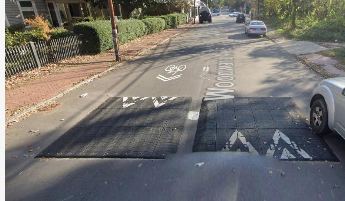
Speed cushions between Deckner Ave and Astor Ave to encourage safety driving speeds.
