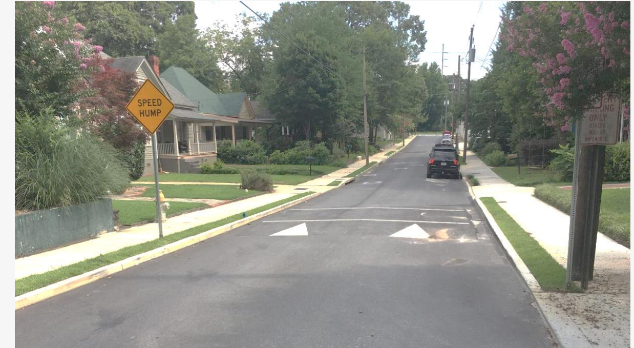
New speed tables for traffic calming
