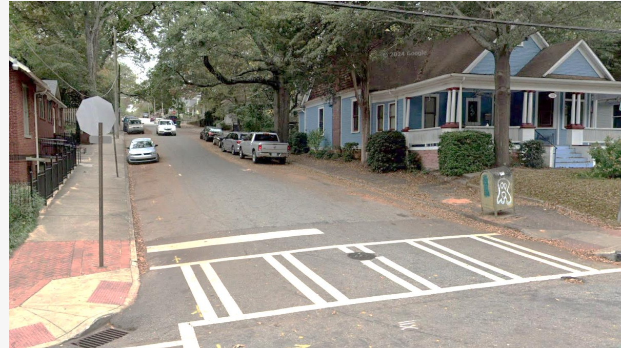
New crosswalk at Glenrose Circle
