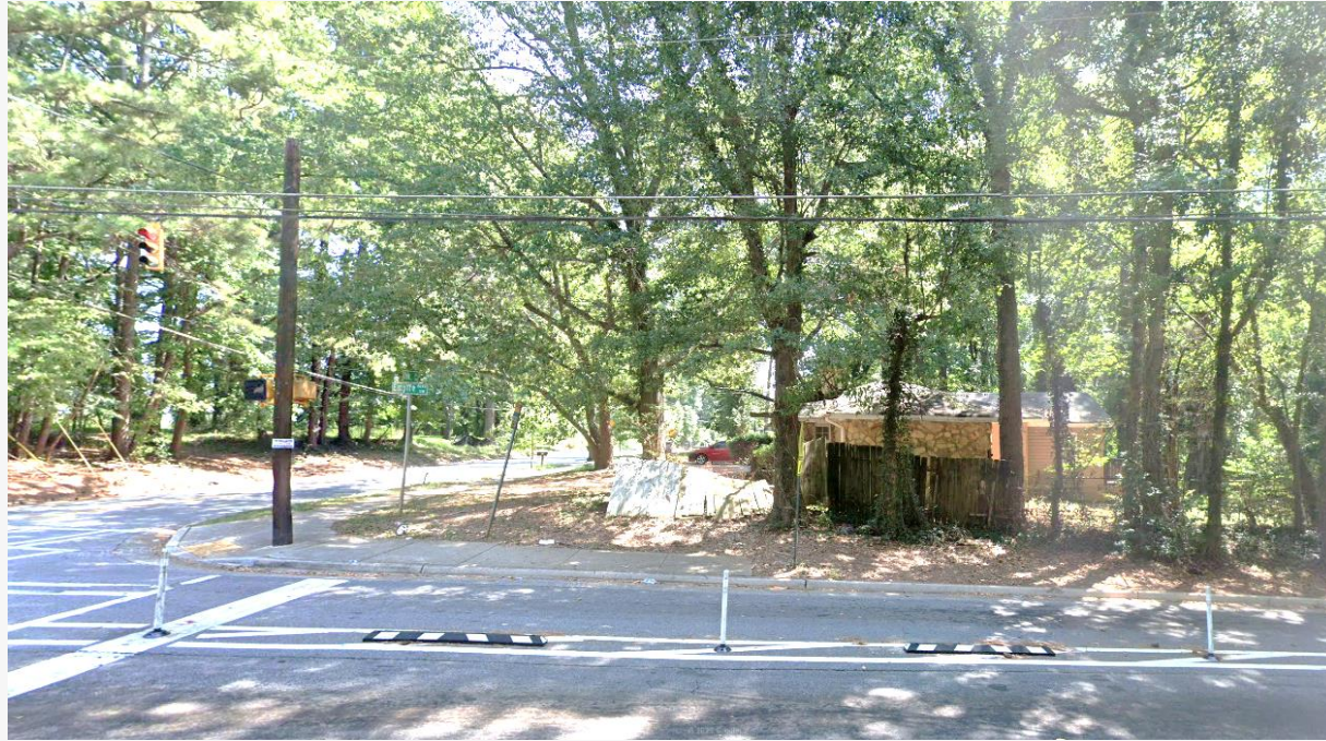
Painted buffer with vertical posts & wheel stops
