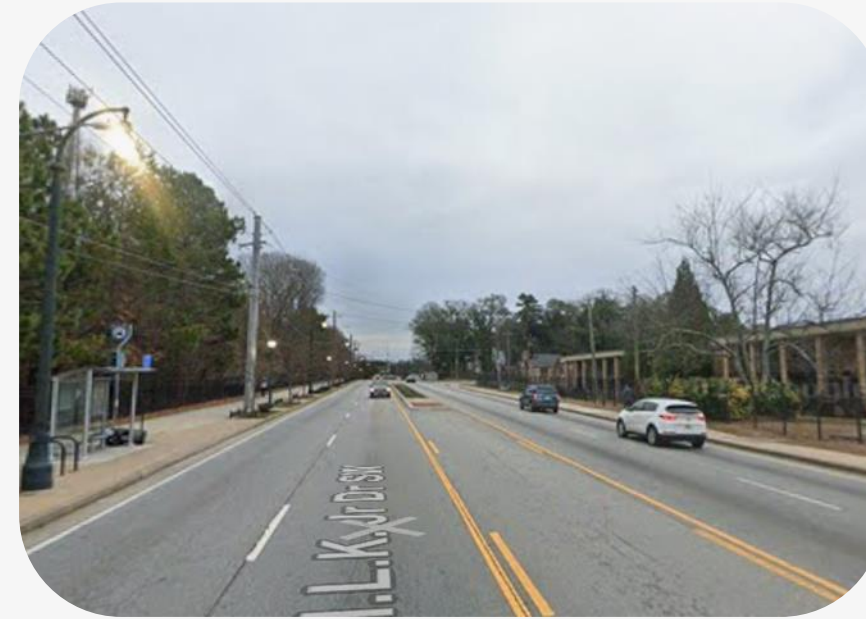
MLK Jr. Drive SW ~20,000 vehicles per day 4 vehicle lanes with center turn lane
