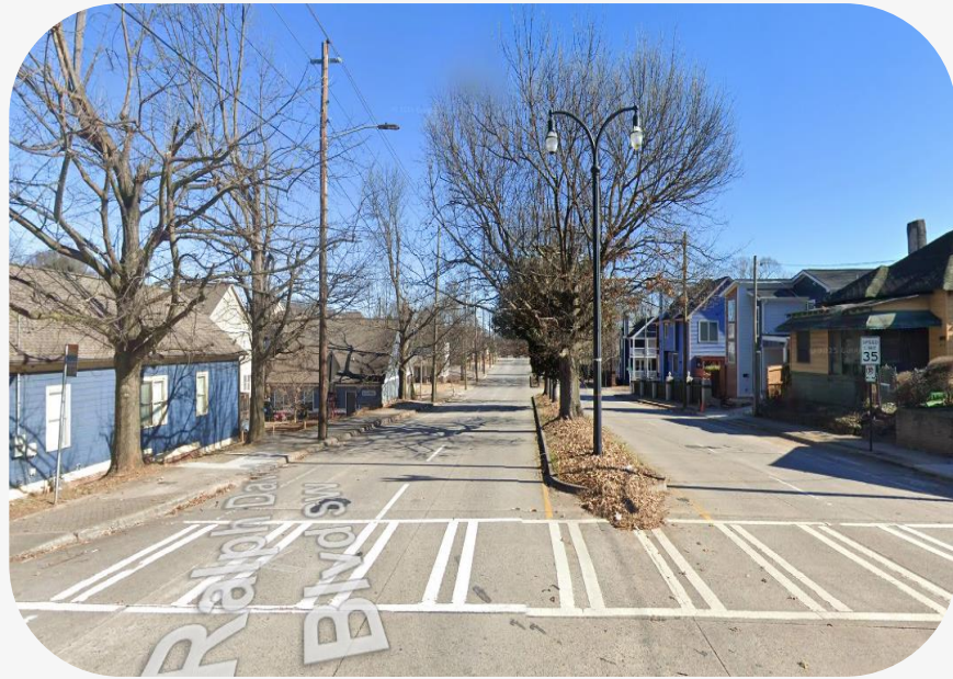
RD Abernathy Boulevard <9,500 vehicles per day 4 vehicle lanes with median and bike lanes
