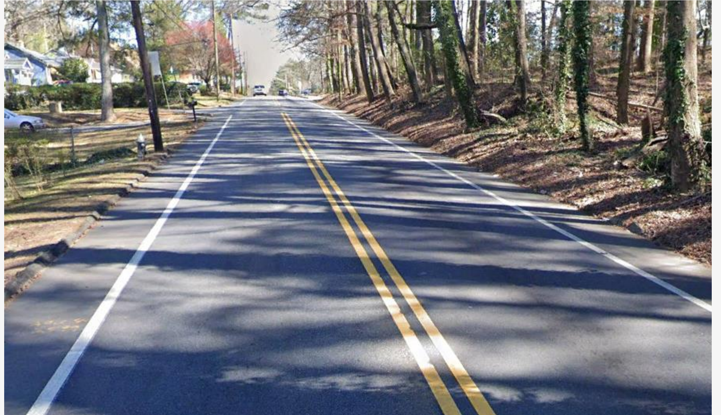
Collier Dr between Simon Terrace & Chilton Dr Looking West
