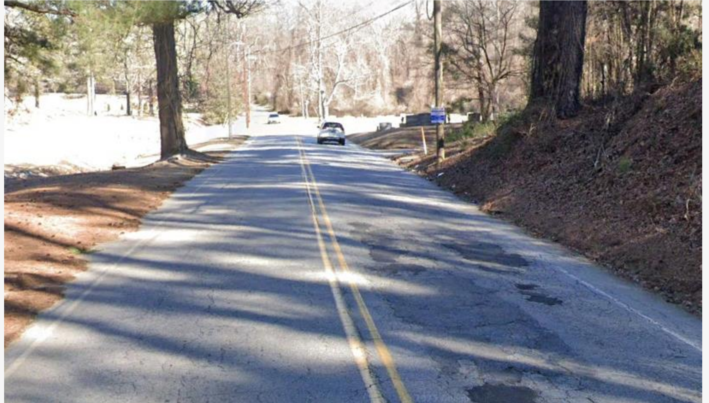
J.E. Boone Blvd between Sewanee Ave & Lincoln Cemetery Entrance Looking East
